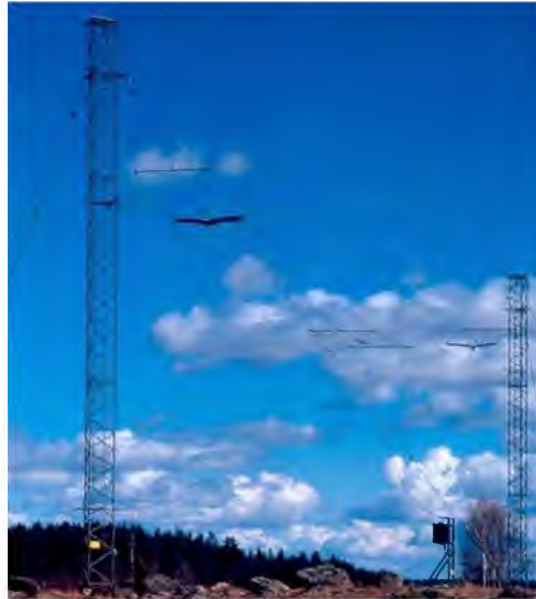
Bredbandsdipol 2 – 9 MHz 10 kW
